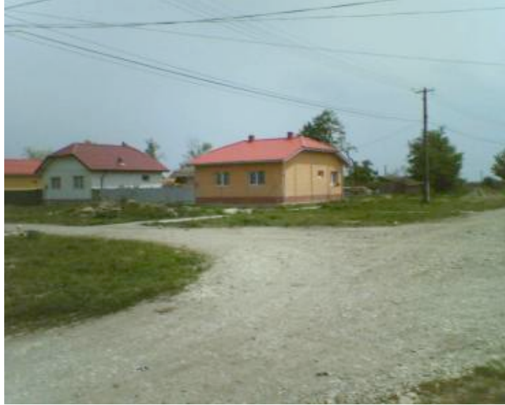
Image 7 – Recently built house after the floods
