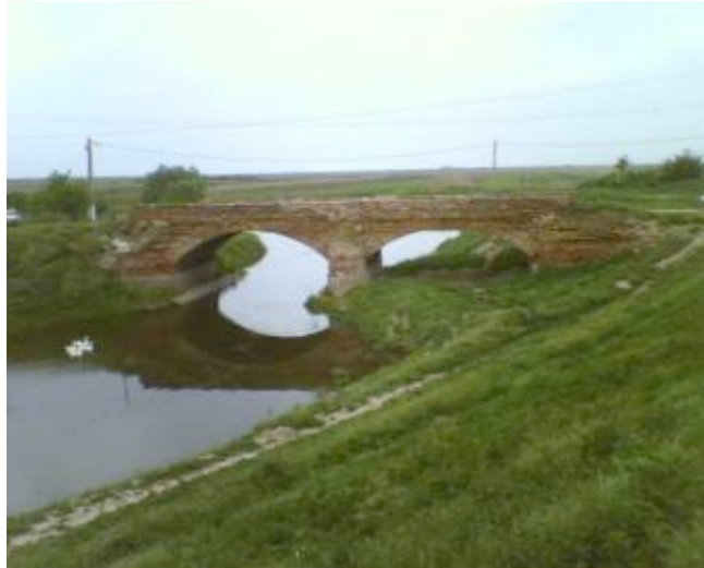
Image 9 – The old brick bridge, present on the list of protected monuments
